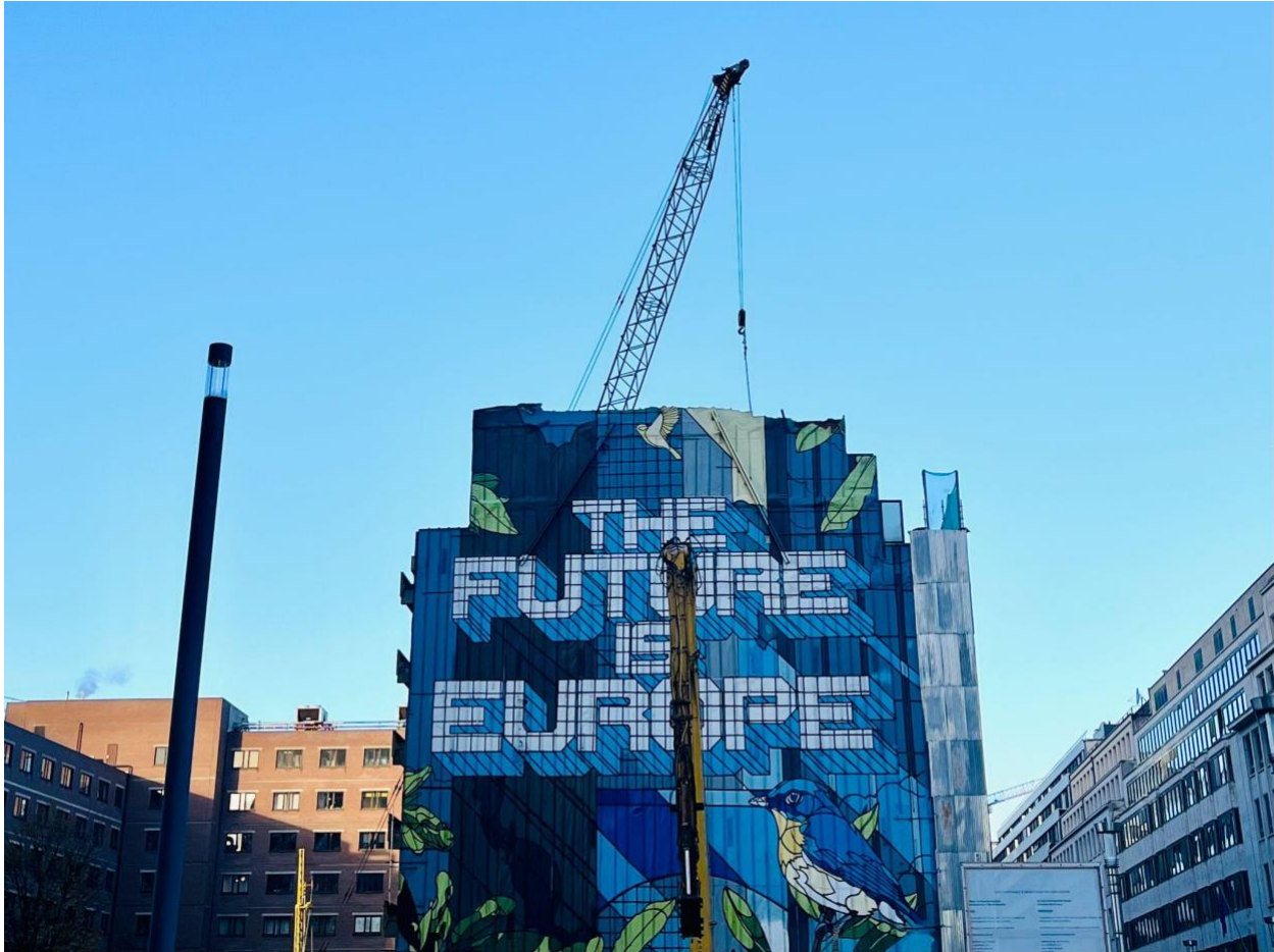
Europe: a work in progress. Photo of Brussels mural 'The Future is Europe' by artist Julien Crevaels, in front of a semi-demolished building and crane in the foreground, by Stephanie Bonnici.
